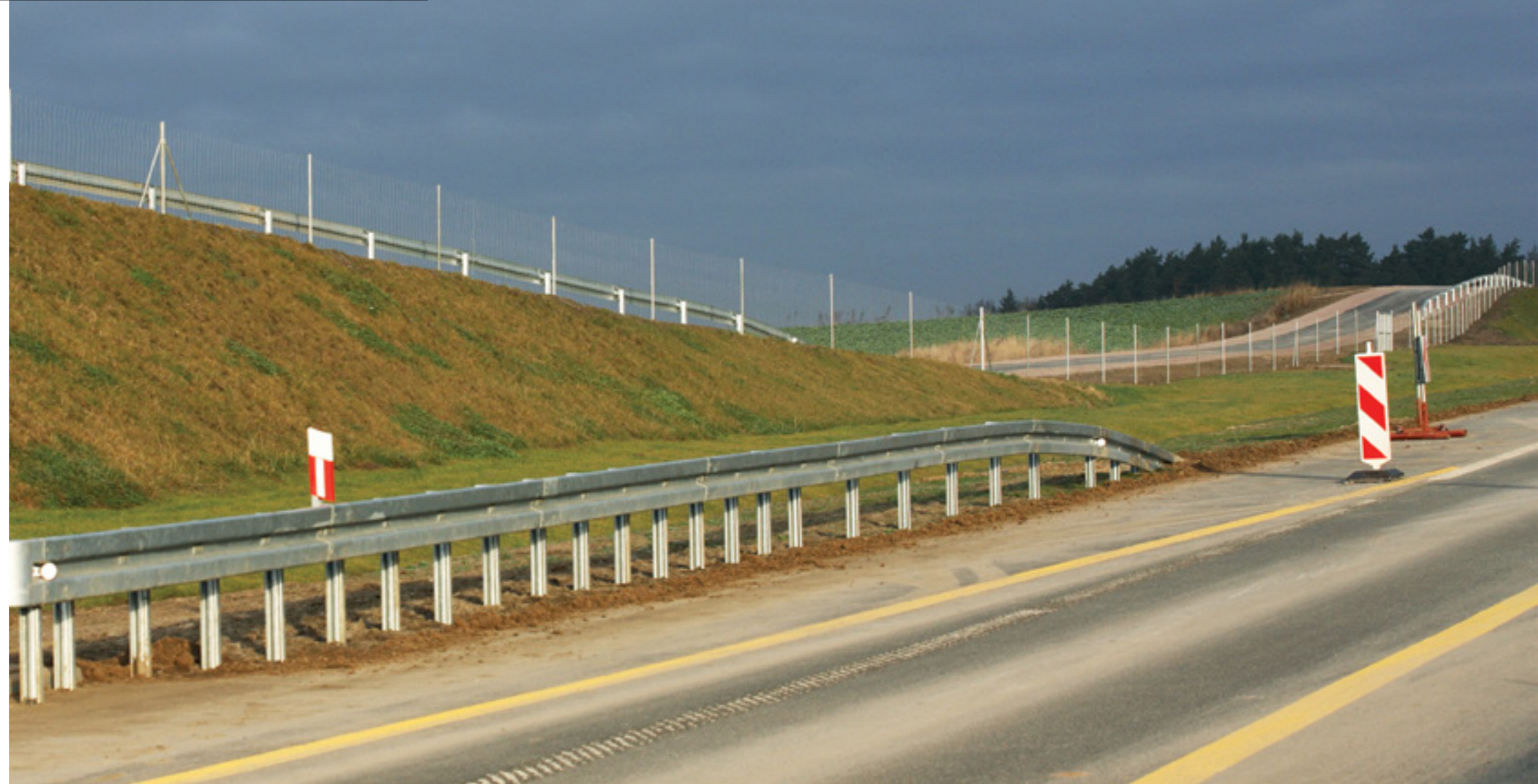
Fencing of the A1 motorway
