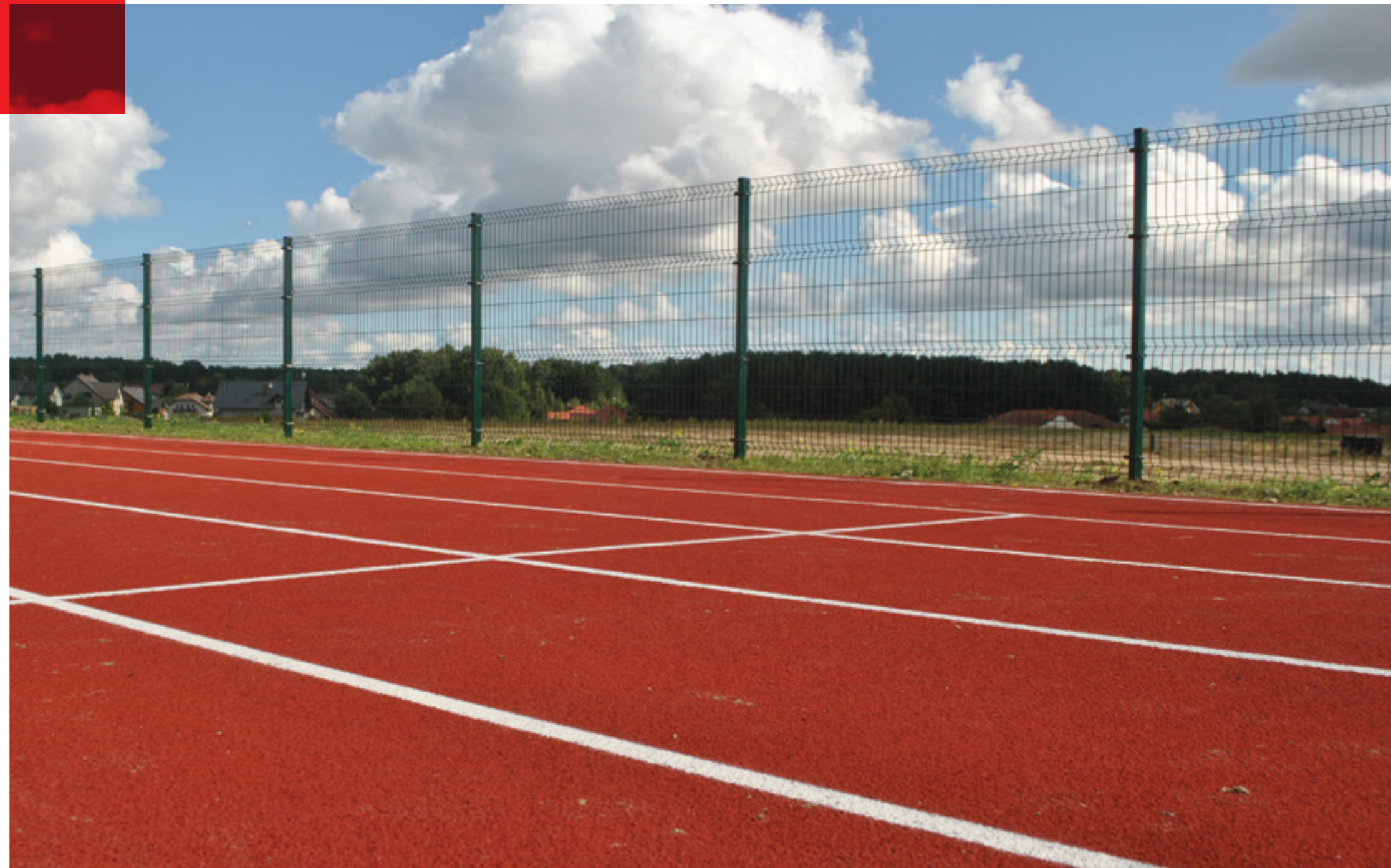
A sports facility fenced with the 3D Ø5 / 5 RAL 6005 H 2030 mm panel
