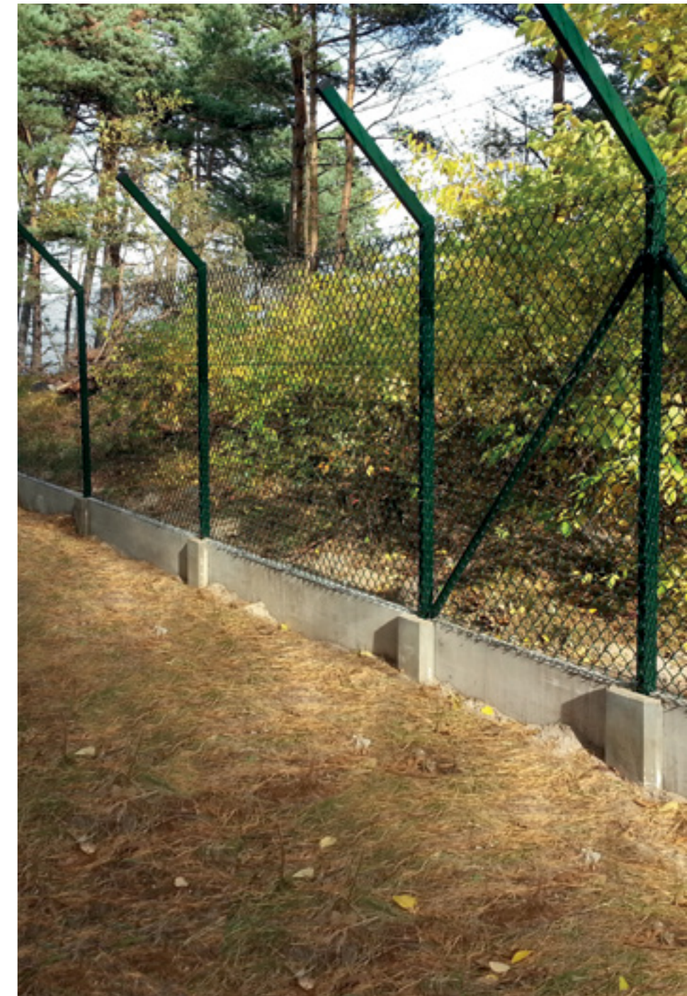
Fencing of a military facility with an increased access control through the use of posts with a single barbed wire angle bracket.
